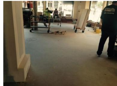
Viking Commercial contracted Dedicated Floors in this challenging tenant improvement project located in the heart of downtown San Diego. After demolition was complete it was discovered that the subfloor was in disrepair. Dedicated determined critical elevations, surveyed the floor and set elevations with a laser, then poured a finished subfloor that was turnkey for the flooring subcontractor. The work was performed in single evening and kept the project moving along at a fast pace.
